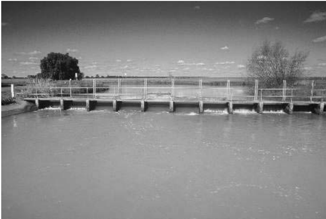
Regulator minor outlet at Waranga basin.
